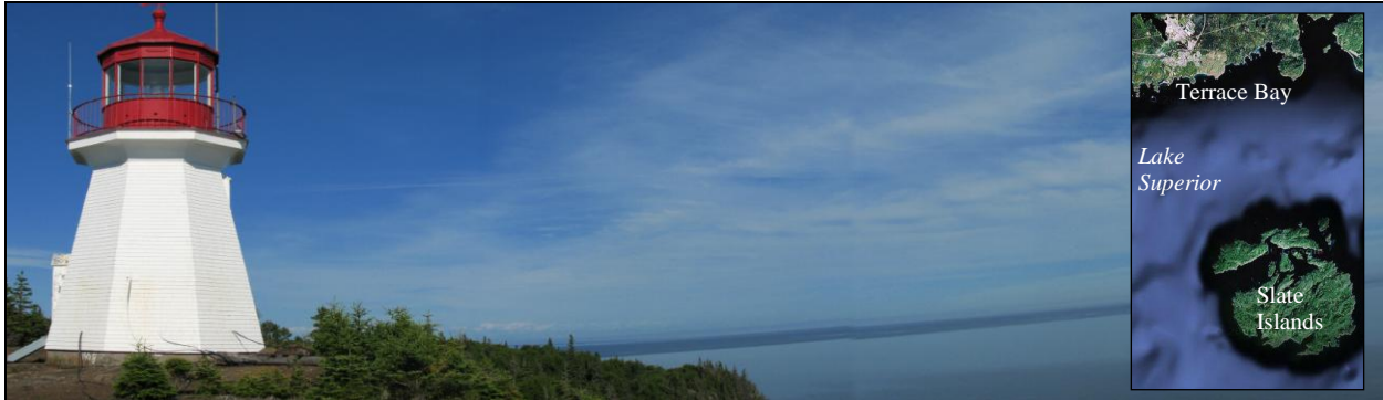
The Slate Islands Lighthouse is the tallest on Lake Superior standing 224 feet above sea level
